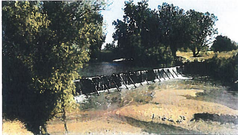
Diversion dam showing boards that can be removed during spawning season.
