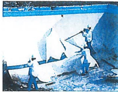
10/18/04: Old fiberglass removed
