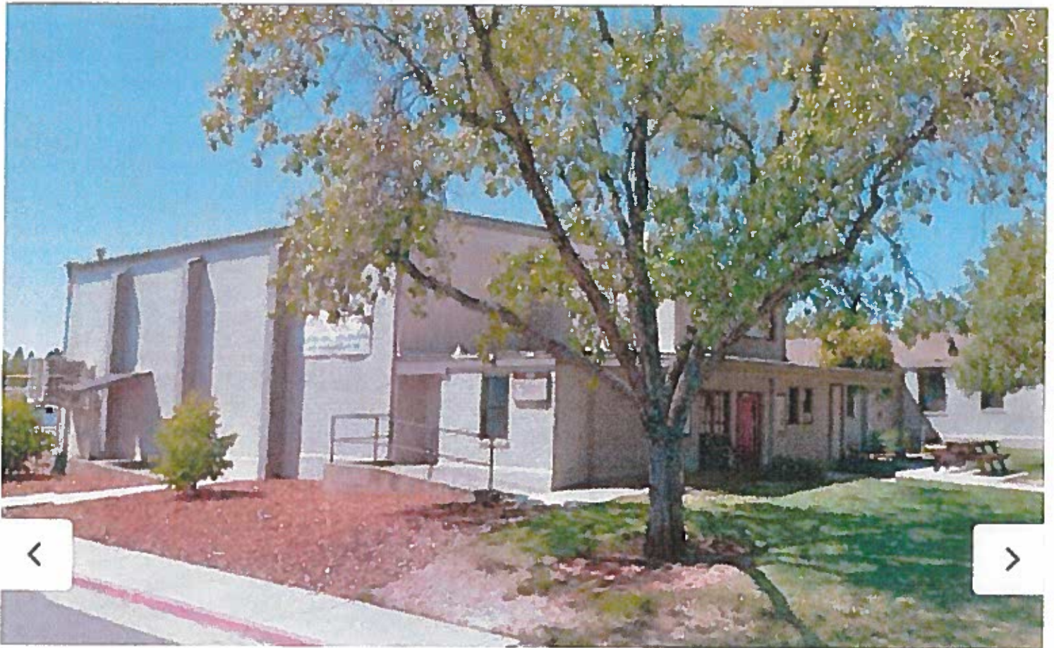
The Dewitt Theater is one of several World War II military hospital buildings at the Placer Government Center that could be torn down. It's not on the affordable housing project footprint.
