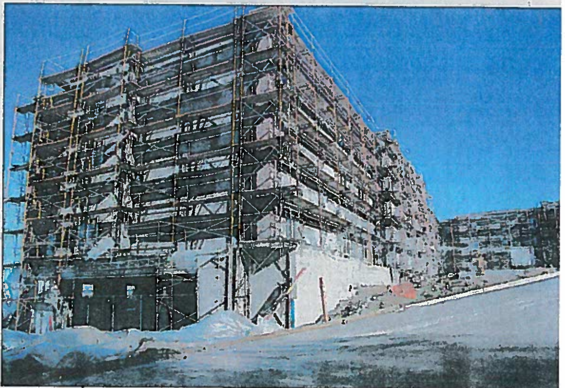
The 128-room Springhills Suites by Marriott on Bowman Road is moving closer to opening as 2019 dawns.
