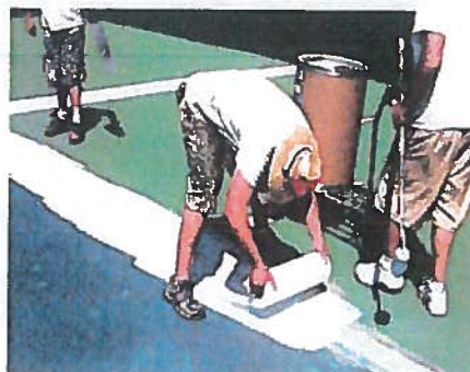
↑ Applying RiteWay Stress Mat
