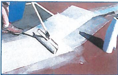
RiteWay Crack Repair System: Laying down micro sealant tape and stress mat.
