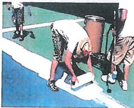
↑ Applying RiteWay Stress Mat
