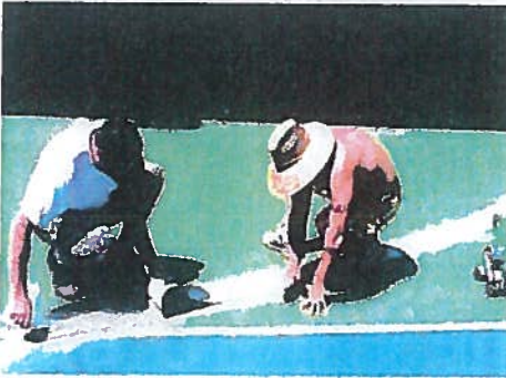
↑ Applying RiteWay MicroSealant Tape
